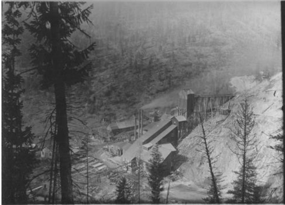
Iron Mountain Mine concentrator located about a mile downstream of Iron Mountain Mine at Pardee 1898
